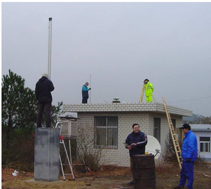
Direct levelling for Jiufeng network between DORIS pier and point 1.
