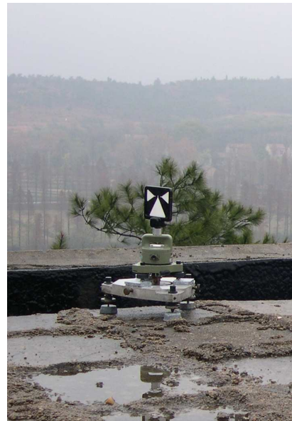
Point 1: platform for temporary point during topometric measurements
